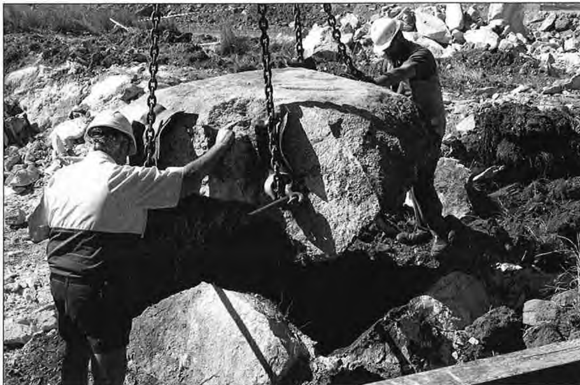
Figure 33 - Block 6 being lifted. Note the tyre-strips protecting the block from the chains.
