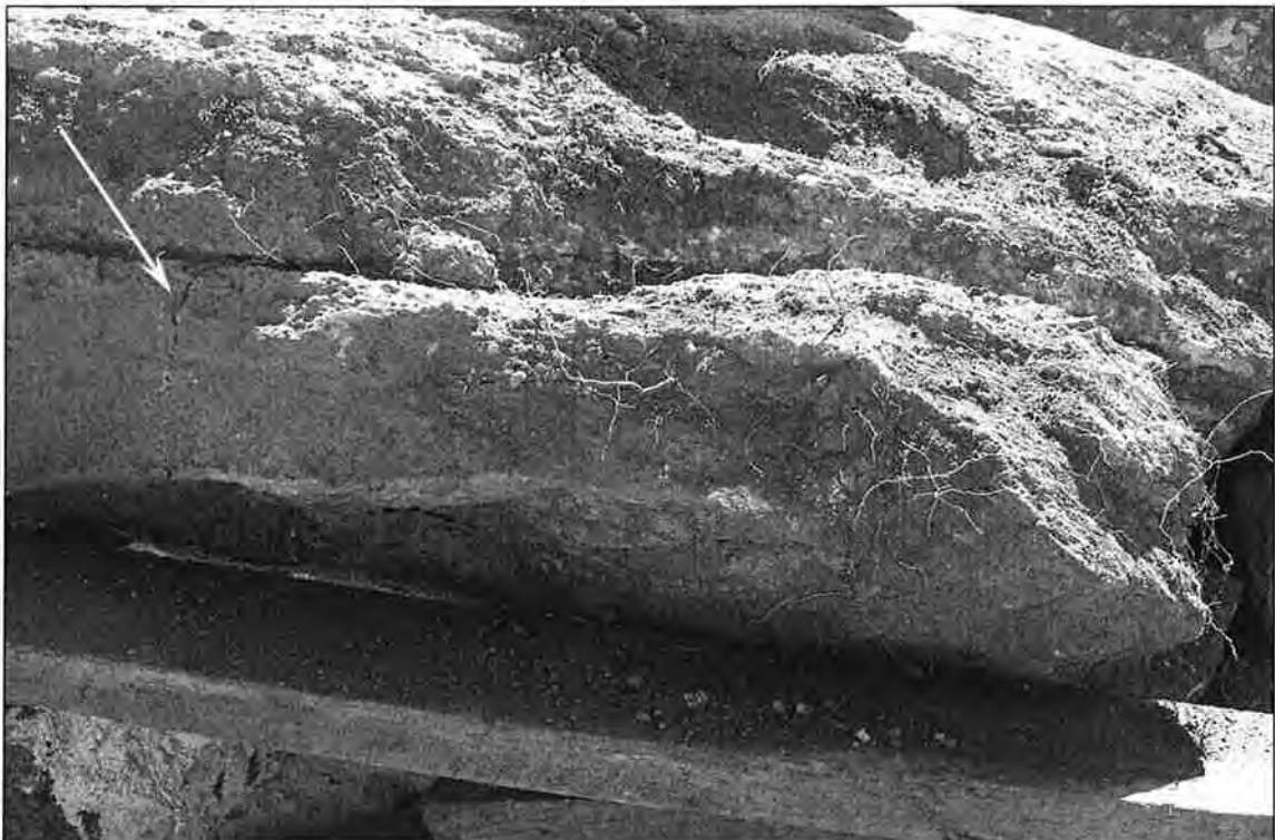
Figure 25 - Close-up of the crack in the lower section of Block 5 prior to removal.
