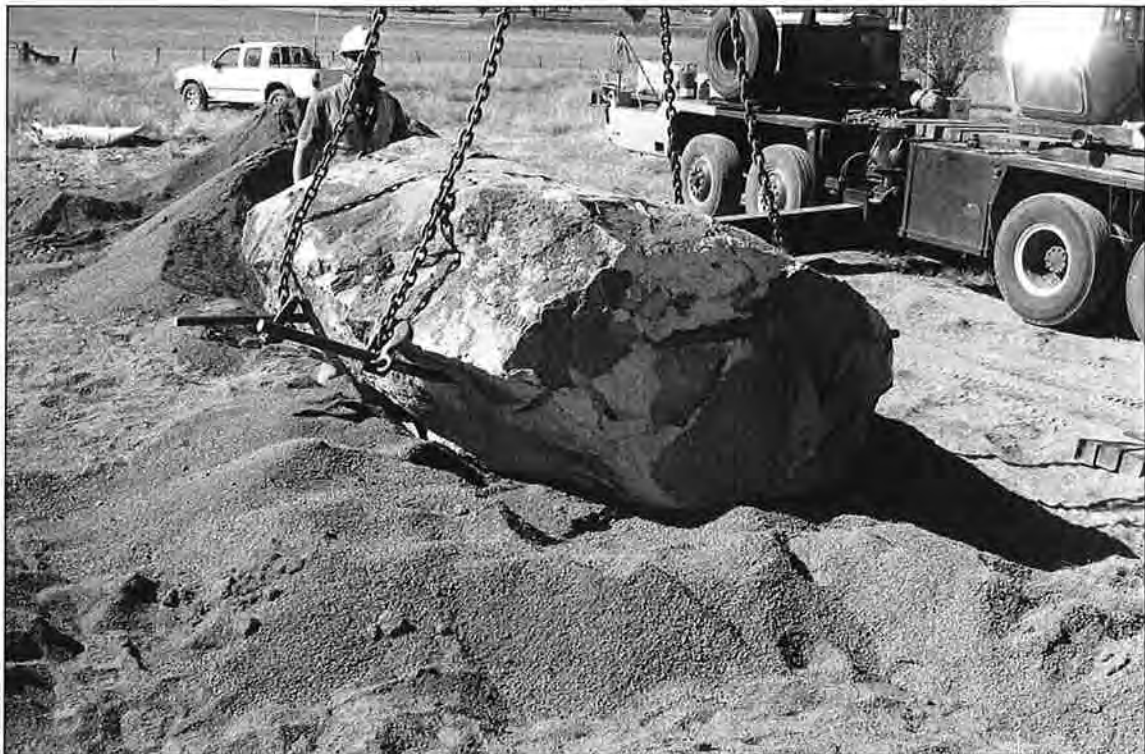
Figure 15 - Block 1 is laid to rest where it will remain until the site is restored and the block relocated.
