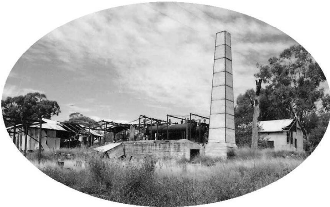
Figure 20 Concrete boiler chimneystack at the Werris Creek Colliery in circa 1970s (McEvilly et al. , 2004)
