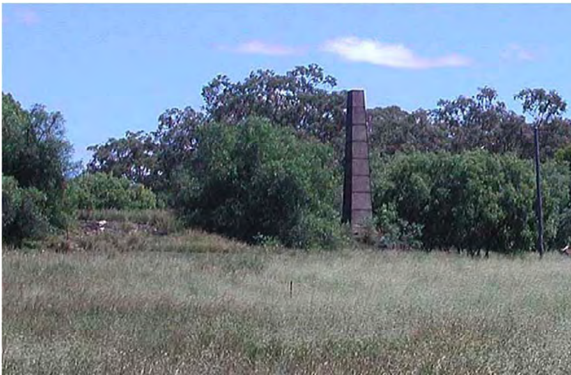
Figure 21 Boiler chimneystack in 2004 (ASR, 2004)
