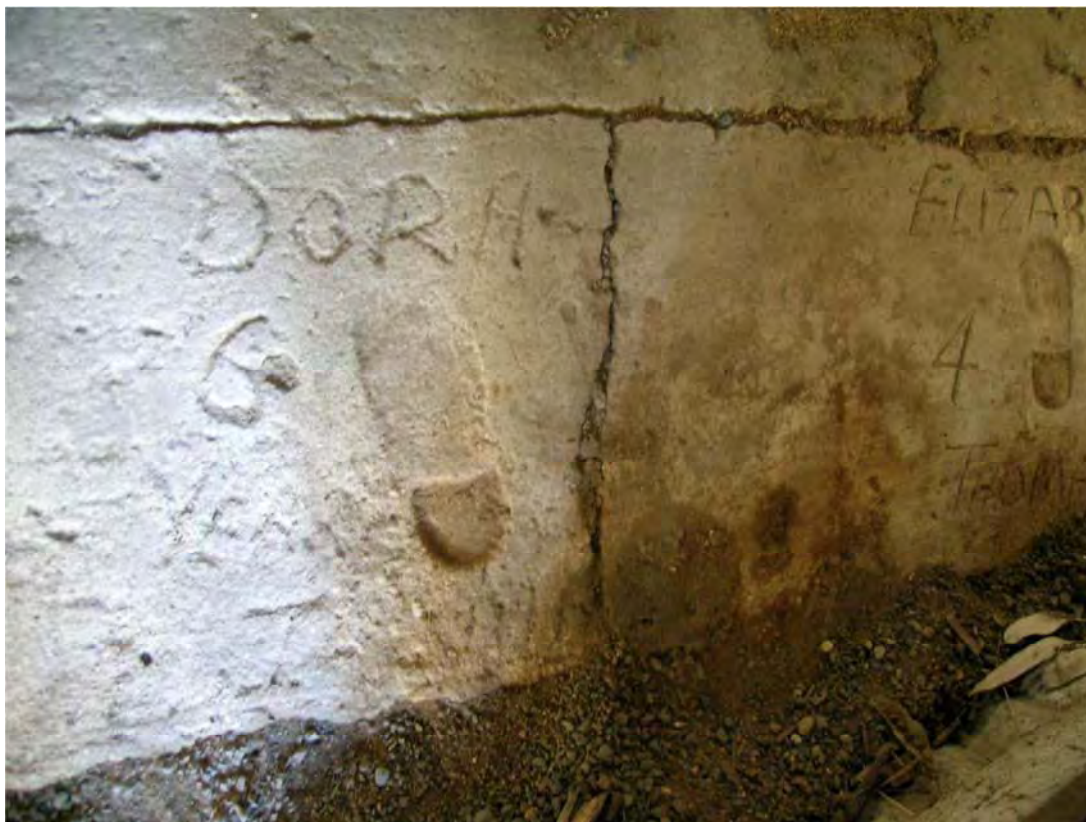
Figure 27 Boot and hand impressions of Deputy Mine Manager's children in concrete slab floor
