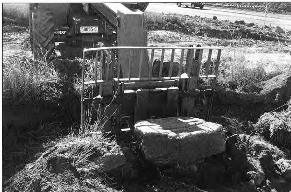
Figure 41 - Block 8 being removed. Note the depth or thickness of the block.
