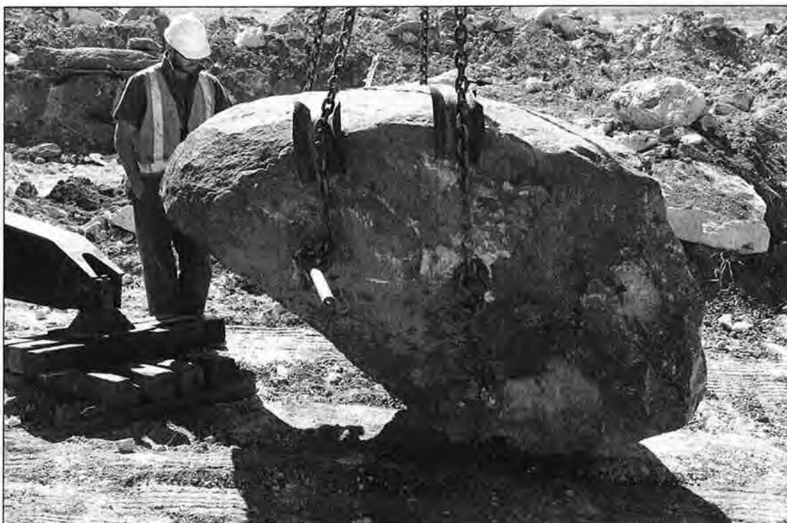
Figure 34 - Block 6 after removal. Note the imbalance caused by the irregular base of the block.
