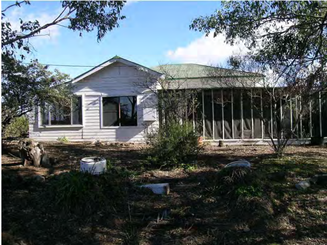
Figure 24 Former Deputy Mine Manager's Residence for the Werris Creek Colliery
