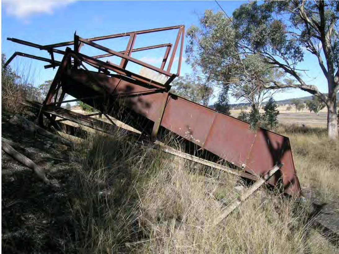
Figure 28 Werris Creek Colliery coal loading chute
