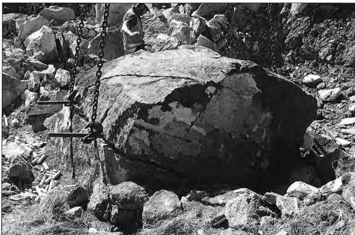
Figure 11 - Lifting bars are in place and the lift begins.
