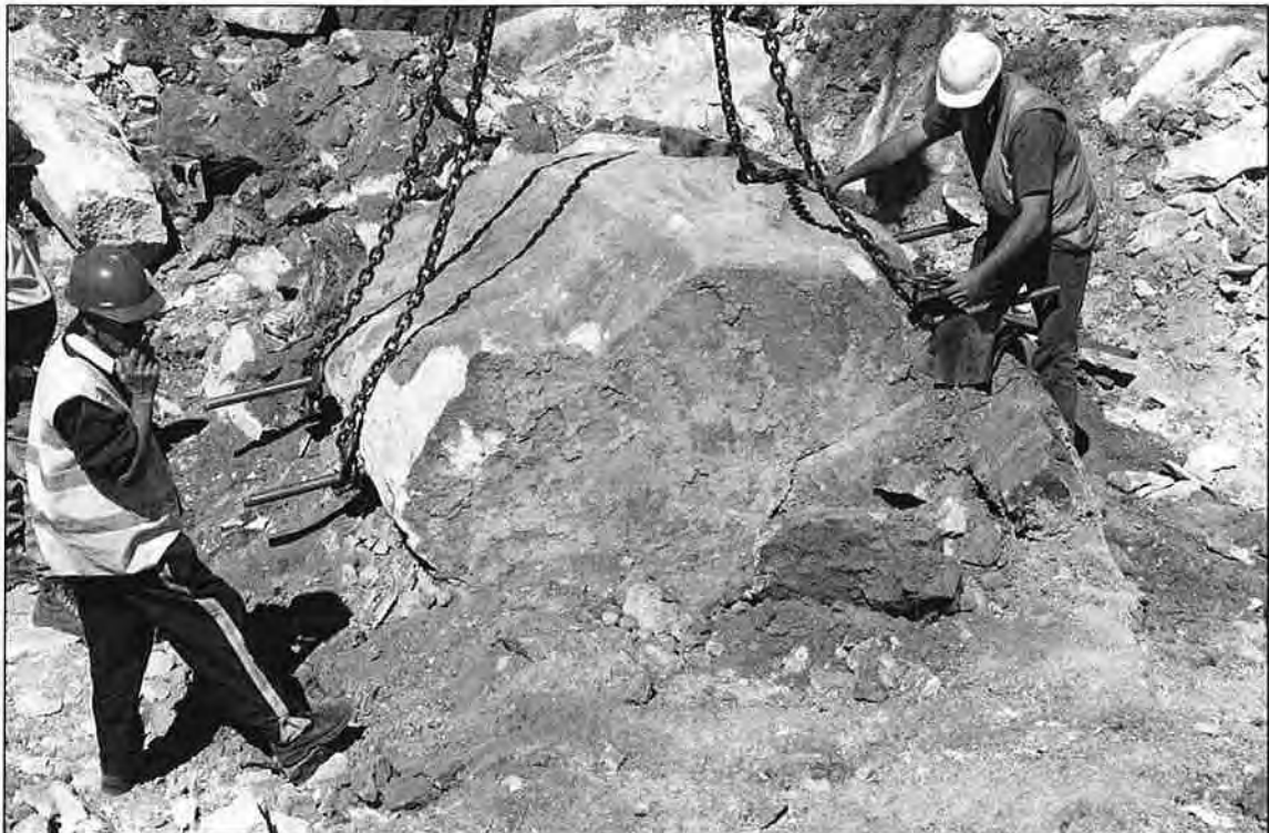
Figure 32 - Block 6 ready for lifting. Note the line of separation between the block and the bedrock.
