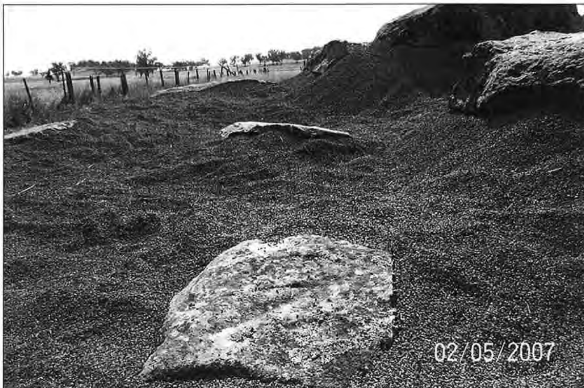
Figure 50 – Crusher dust has built up around the blocks to retain the ground moisture (photo. Rob Snook)
