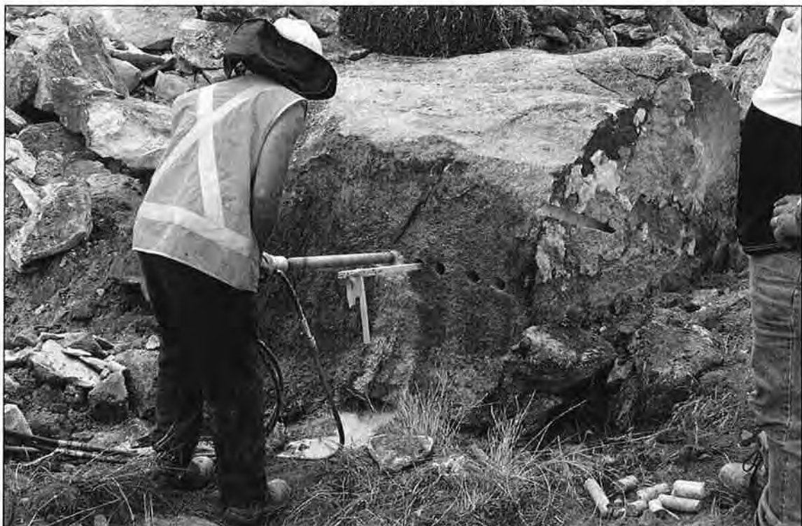
Figure 7 - Drilling a series of deep holes to create a plane of weakness.
