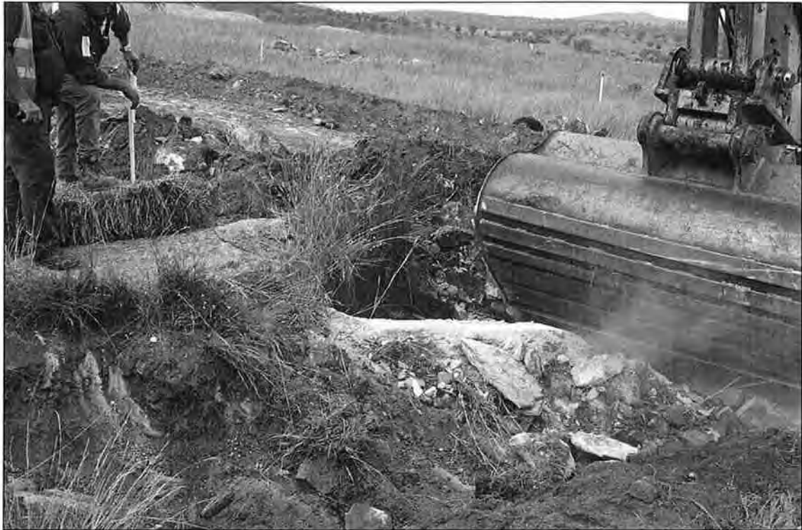
Figure 6 - Removing the surrounding bedrock to expose the sides of Block 1. The straw bale is protecting the grooves.
