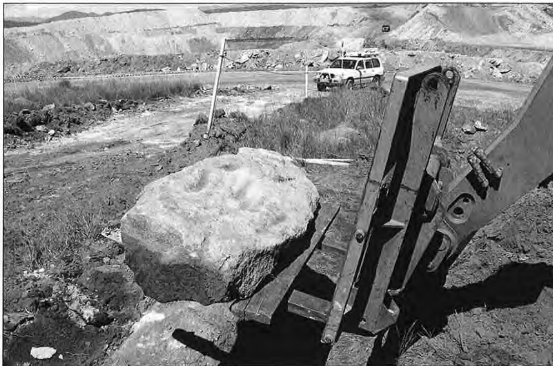
Figure 21 - Block 4 is removed by forklift.
