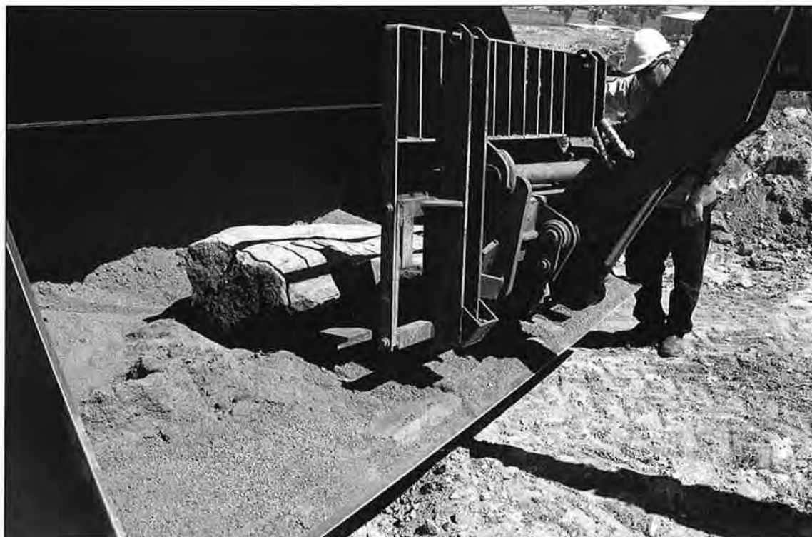
Figure 22 - Block 4 is lowered onto a bed of crusher dust for transportation to the storage area.
